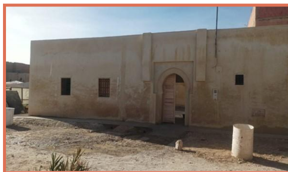
Main façade: Traditional plastering, main door, and windows.
