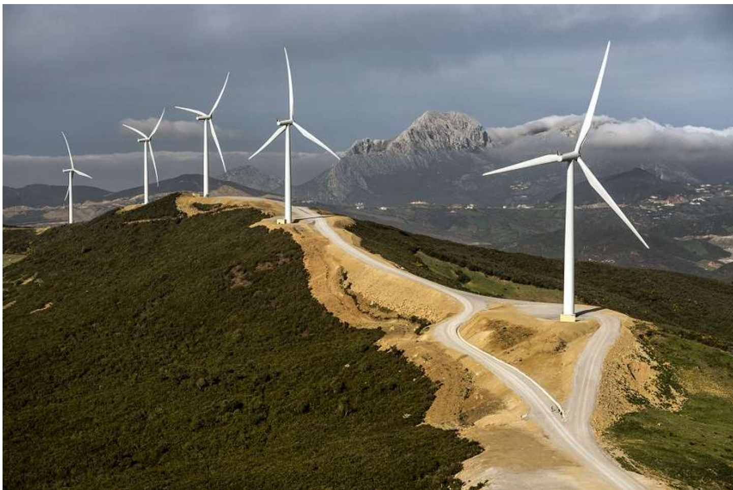
The Haouma wind farm. Photo provided by Siemens Gamesa Morocco.
