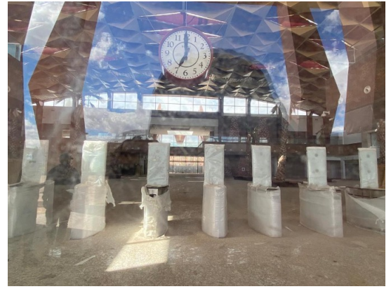
Figure 08 The Electronic Gates in Azzouzia Station.
