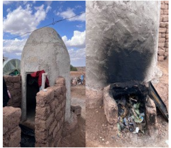
Figure 13 A small hammam constructed by villagers. They lit trash and wooden sticks to light a fire.
